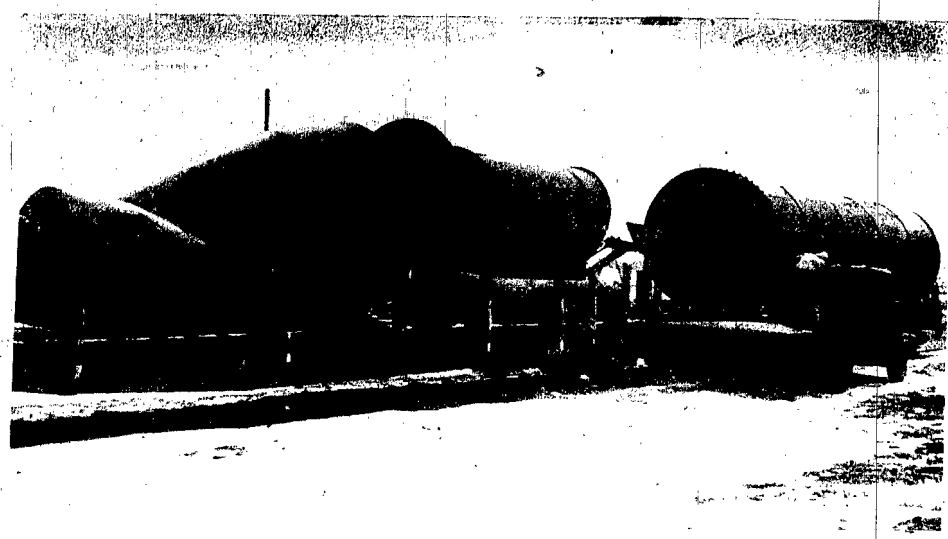
CONSTRUCTION OF THE WINSIDE DEHY, INC., took a big step forward this week as most of the mechanical end-of-the plant was unloaded in Winside. Still on the flatcars in this photo are, left to
